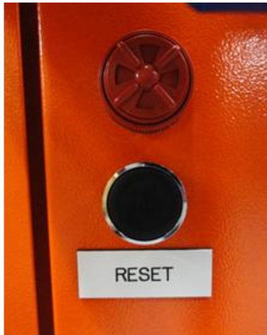
Figure 3-6: CCM Status Indicator audible alarm
