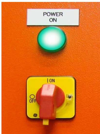
Figure 1-13: Main Power Disconnect
