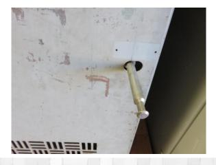
3. Slide the ArcSafe cutting template over the interlock, as shown, and ensure the tab on the right side of the template is flush with the right-side of the switchgear.
