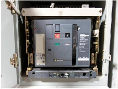
2. Remove the charging handle adapter from the RSA by removing the quick disconnect clevis pin. This will be re installed later.
