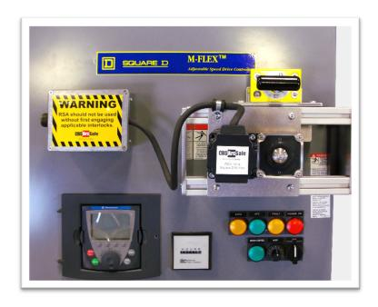
**Step 5:** Next, find a suitable place to mount the motor control box. The motor control box is mounted using the magnet on the underside of the box. The box should be located in a location where it will not interfere with the remote operation of the MCCB.
