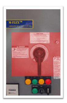
**Step 2:** Next, ensure that the handle operator on the RSA-161A matches the location of the handle to be remotely operated. If it does not, jog the handle to the correct position either manually or the RSO control device.
