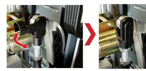
8. Manually push the charging arm back to its resting position before beginning operation. The RSA is ready for remote operations.
