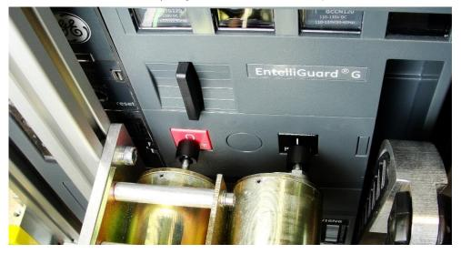
6. Place the charging arm adapter, removed in step 2, over the charging arm of the breaker. To do this pull out the charging arm slightly and slide the adapter over the arm.
