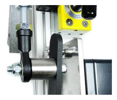
5. With the breaker handle and RSA operator arm fully in the DOWN position, slide the travel stop up until it contacts the arm as shown, and tighten the bolt.
