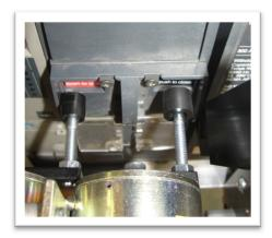
**Step 4**: Next, pull the charging arm out away from the breaker and place the black composite handle adapter over it. Press the adapter onto the changing arm until it fits firmly and completely over the charging arm as shown to the right.
