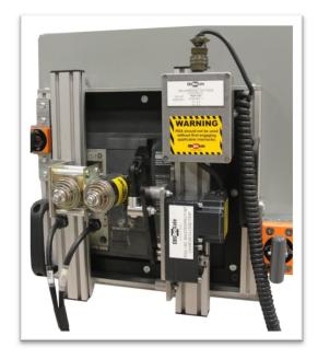
**Step 3**: Next, verify that the two solenoid plungers are properly aligned with the CLOSE and TRIP buttons as shown on the figure to the right. If they are not, adjust the location of the solenoids until they are properly aligned. The recommended distance from the plunger to the pushbutton is 1/8".
