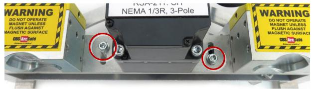
3. With the breaker in the ON position, slide the ON travel stop so it contacts the actuator arm, and tighten the bolt.
