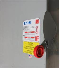
2. Slide the RSA over the switch handle, and ensure the RSA handle adapter fits properly over the breaker switch.
