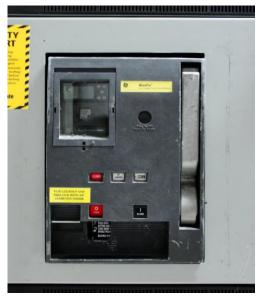
2. Remove the charging handle adapter from the RSA by removing the quick disconnect clevis pin. This will be re installed later.
