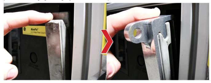
7. Reconnect the charging arm adapter to the RSA-120 using the clevis pin from step 2.
