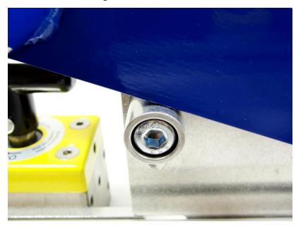
5. With the breaker handle and RSA operator arm fully in the DOWN position, slide the travel stop up until it contacts the arm as shown, and tighten the bolt.
