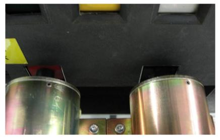
6. Place the charging arm adapter, removed in step 2, over the charging arm of the breaker. To do this pull out the charging arm slightly and slide the adapter over the arm.
