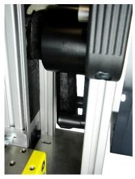
6. To attach the RSA to the breaker turn the handles of the twist-lock magnets 180° clockwise. The RSA is now ready for remote operation
