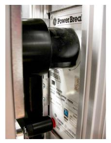
4. Ensure the locators on the RSA are properly positioned, and seated flush against the operating handle housing, as shown.
