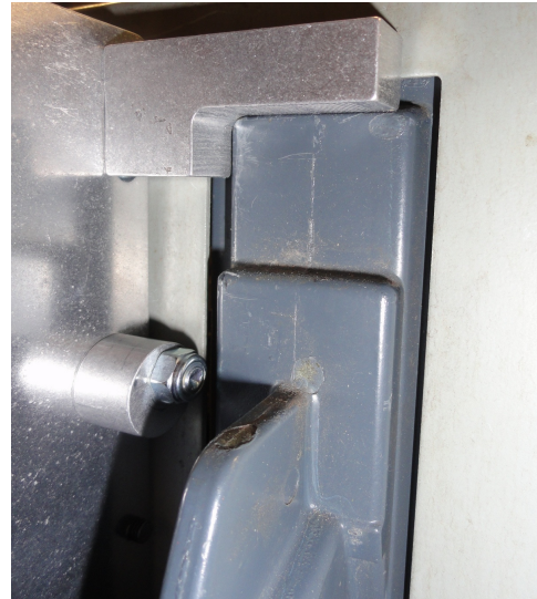
Step 4: Ensure the top support of the RSA-99 is positioned against the top of the switch.
