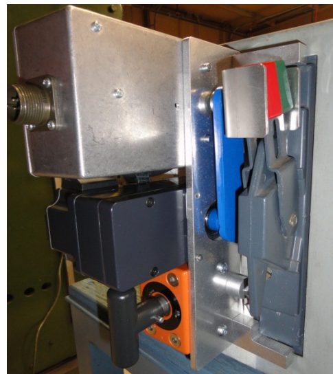
Step 6: The RSA-99 properly installed on the switch and is ready for operation.
