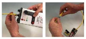
**STEP 4:** Carefully position the PB-16 over your button, hold the magnet firmly against the switchgear door, and the rotate the magnet lever clockwise to the ON position.
