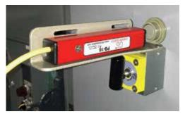
The magnet should be firmly against the switchgear door. If the magnet is not set firmly against the door, it will likely not have enough holding power to stay on the door when actuated.
