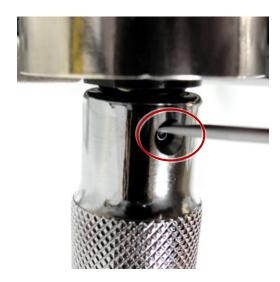
2. On the de-energized and OPEN test breaker, extract the breaker's racking handle, and fit the racking adapter to the handle as shown in the Installation section of this manual.
