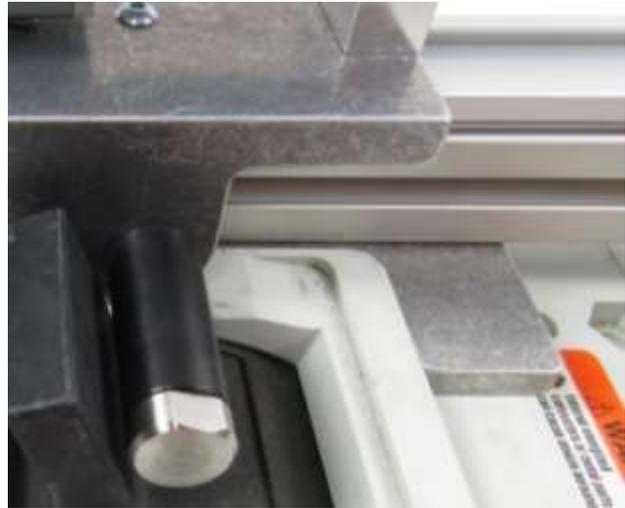
3. Secure the RSA to the breaker by rotating the two twist-lock magnet handles clockwise until the RSA is securely in place.
