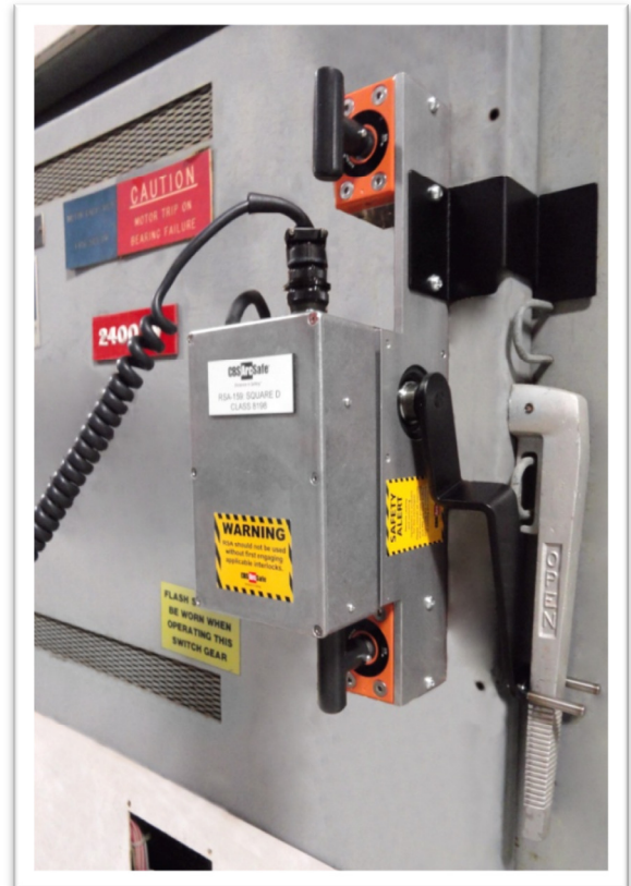
Figure 2: Slide the RSA-159 handle locator over the handle operator on the breaker
