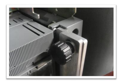
Step 5: Lastly, ensure that the solenoid pushbutton operators have not moved and are aligned with the breaker's pushbuttons. The RSA-174E is now ready to operate.
