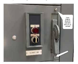
**STEP 2:** Prior to installing the RSK-ABL1 actuator, verify that the magnets are in the OFF position. Start with the RSK-ABL1 held low on the switch and while lifting up on the operating handle with your fingers, slip the actuator arm under the operating handle and move the up and over the operating handle mechanism.
