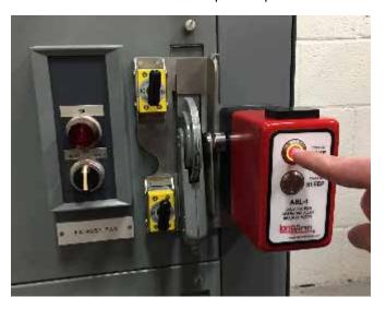
**STEP 2:** While standing at a safe distance, press and hold the ENABLE button on the hand-held controller. The yellow light should illuminate. Then press and hold the button corresponding to the handle direction that is desired (ON or OFF). Both the ENABLE button and the ON or OFF button must be held simultaneously until the full stroke of the operating handle is complete. Then the buttons can be released and the actuator will return to its neutral position.
