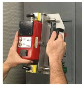
**STEP 3:** With actuator now flush against the MCC door, twist the magnet levers on both magnets one-half turn clockwise to lock the magnet and actuator in place.
