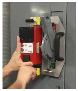
**STEP 4:** For the wireless versions of the RSK-ABL2, the installation is complete and it is ready to operate. See Section 4.2 for the operating procedure.
