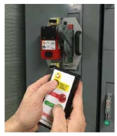
**STEP 3:** When completed with operating the RSK-ABL2, power the actuator OFF by pressing the SLEEP button.
