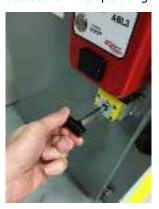
**STEP 3**: Disconnect cable (for cabled versions only) and return components to carrying case or store on the side of the MCC. (See Section 5.0 for details)
