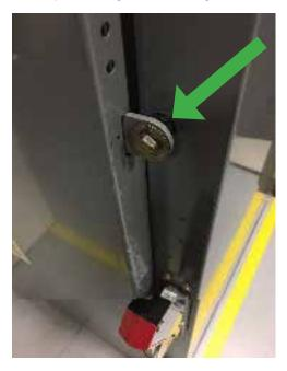
**STEP 2:** Prior to installing the RSK-ABL3 actuator, verify that the magnets are in the OFF position. Start with the RSK-ABL3 held low on the switch. Slip the actuator arm under the operating handle and move the up and over the operating handle mechanism.
