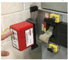
**STEP 6:** When ready to operate the disconnect handle on the MCC, stand at a safe distance from the MCC, press and hold the ENABLE button on the hand-held controller, and rotate the control switch to the desired position - ON or OFF. Hold the ENABLE button and the control switch until the RSK-CHL1 moves
