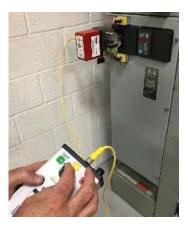
the MCC operating handle the full distance required. Release the ENABLE button and control switch once the MCC operating handle has reached full stroke.
