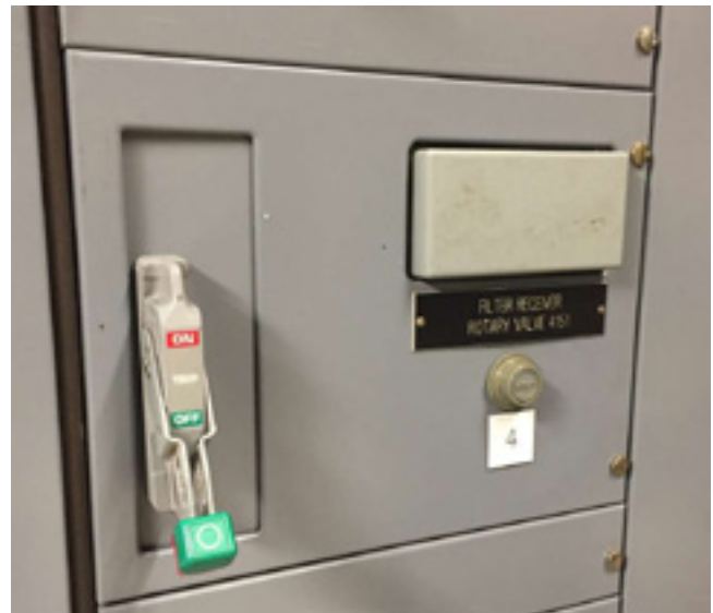
This is a typical switch that the SDL6 is intended to operate.
