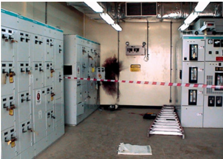
March 4, 2009, at the Jubail Project in Riyadh, Saudi Arabia: Three workers were removing a 480-V molded-case circuit breaker from the bucket of an energized motor-control center (MCC) when an electrical arc flash occurred, severely injuring them. All three sustained first- and second-degree burns and were hospitalized following the accident.
